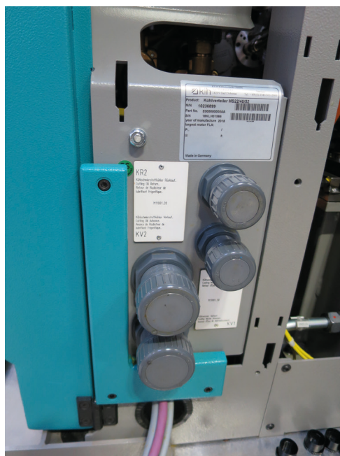
Illustration 01: cooling water connections at a multi-spindle machine
